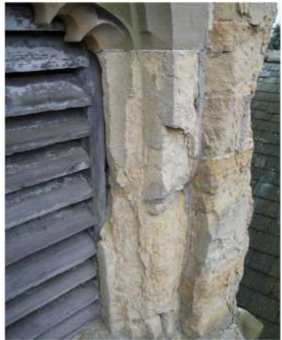
Tower masonry was in a poor and fragile state. Stones had lost considerable section. Ashlars and quoins were considerably decayed. Reveals in the belfry louvres were so badly decayed that frame sides were gapped.
