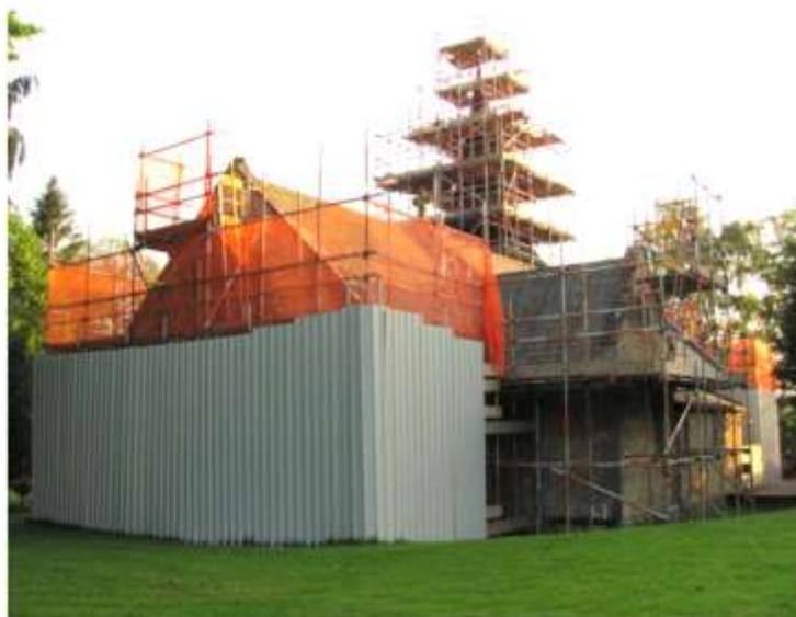
Masonry work started, removing damaged ashlar and quoins, working new ones and replacing them – this work was ongoing throughout the project.
