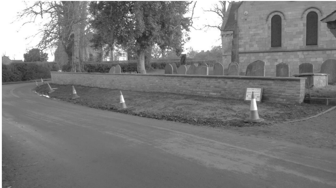
The newly completed wall
