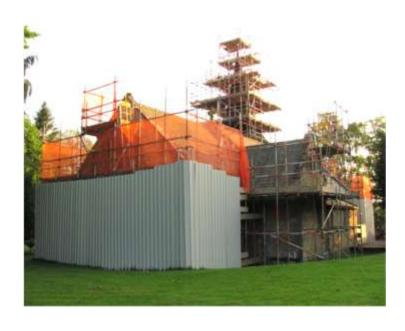
Masonry work started, removing damaged ashlars and quoins, working new ones and replacing them – this work was ongoing throughout the project.
