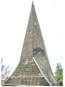
The spire had been damaged by woodpeckers trying to dislodge insects from under the shingles and felt covering which had left numerous large holes in the felt, some down to the broaches and others through to the timbers. Felt had worn through or was ripped and had totally deteriorated in places. Shingles were missing and others ripped. Water was getting into the building. In addition there were holes in the gutter with water leaking onto the tower back gutter and the fall pipe was cracked.
