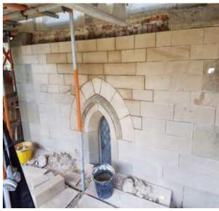
All ashlar replacements were completed to the nave west gable, vestry and chancel. 42 extra ashlars were replaced to complete the replacements to the edge of the window hoodmoulds.
