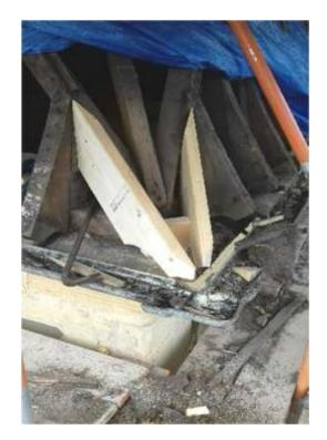
July saw the continuation of masonry works and the start of some roofing works. The core of the masonry indicated the poor state of all elevations and it was deemed the core to all elevations required consolidation.
