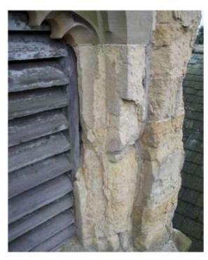
Tower masonry was in a poor and fragile state. Stones had lost considerable section. Ashlars and quoins were considerably decayed. Reveals in the belfry louvres were so badly decayed that frame sides were gapped.
